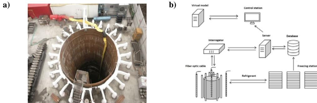
Fig. 1. (a) freezing system (the diameter is 10 m); (b) structural diagram of monitoring system.
